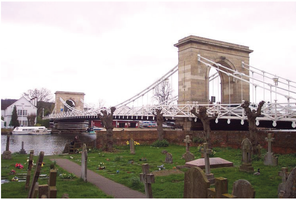
Abb. 3: Kettenbrücke in Marlow, Buckinghamshire. Fotografie von Christopher J. Wood, 2004. URL: https://commons.wikimedia.org/w/index.php?title=File:Uk-marlow-bridge.jpg&oldid=151252453&uselang=de
